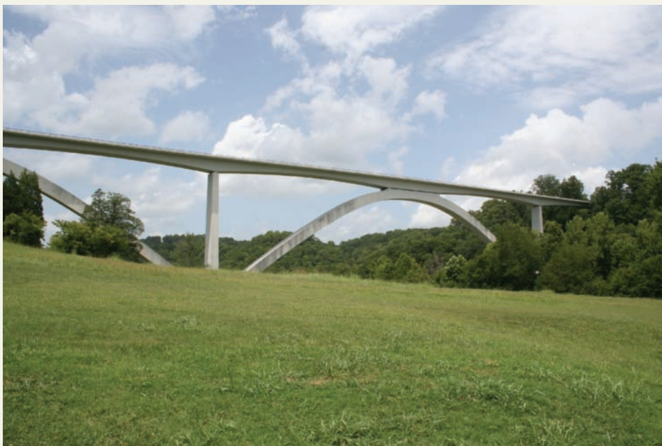
The Natchez Trace Parkway Bridge, in Williamson County, Tennessee, is a concrete double arch bridge. The unique open design of the bridge places strict strength requirements on the concrete used. The weight of the bridge is concentrated at the crown of each arch. National Park Service
